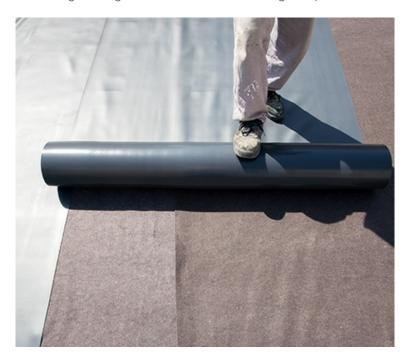
GCP Applied Technologies proposed BITUTHENE®3000HC, an adhesive membrane that is chemically resistant and provides superior protection against aggressive soils, ground water, methane, carbon dioxide and radon gases. BITUTHENE®'s twin seal overlap system ensured highest waterproofing integrity and protection for the lifetime of military architecture.
