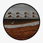
Most structures, especially those on piled foundations, are liable to partial or full ground settlement below the slab. When ground settles or compacts unbonded membranes will fall away from the structure leading to failures and water penetration.
